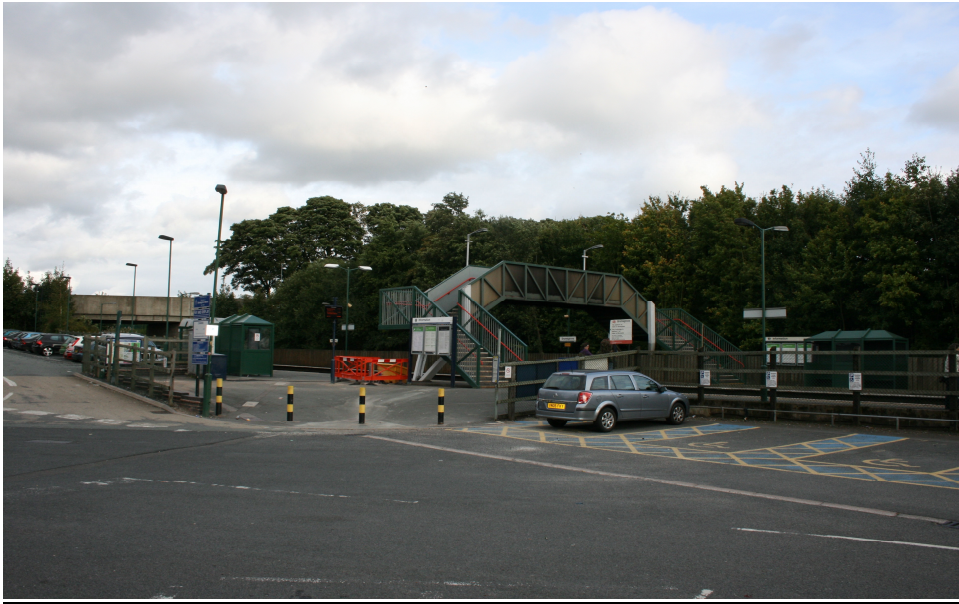
Figure 10: Bromsgrove Train Station
